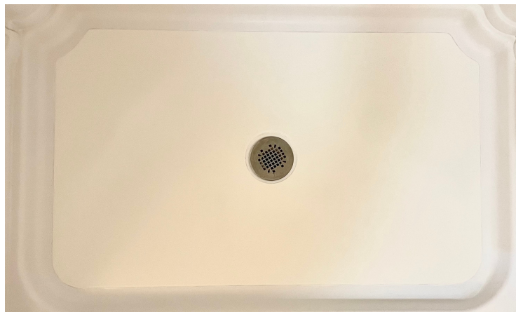
COMPLETED SHOWER INSTALLATION
