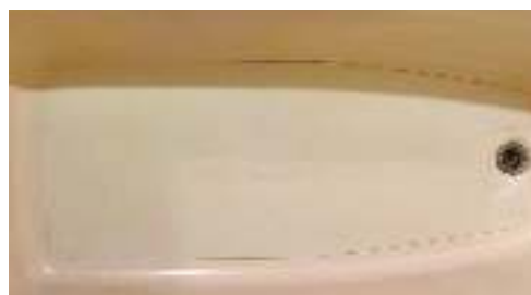
DRAIN WRAP INSTALL
