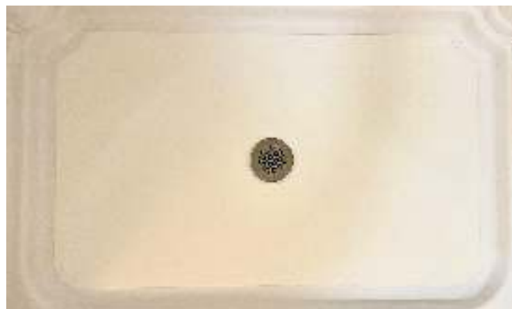
COMPLETED SHOWER INSTALLATION
